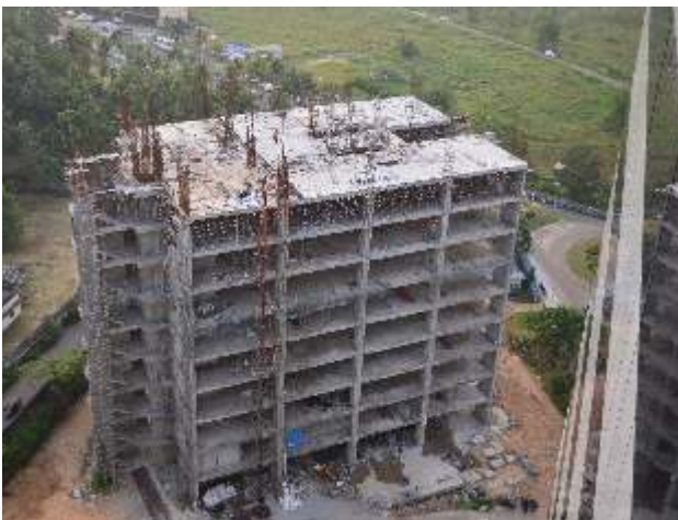
Caspian Tech Park- Work in progress
