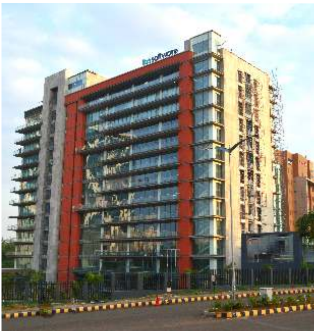
IBS Campus-Nearing Completion
